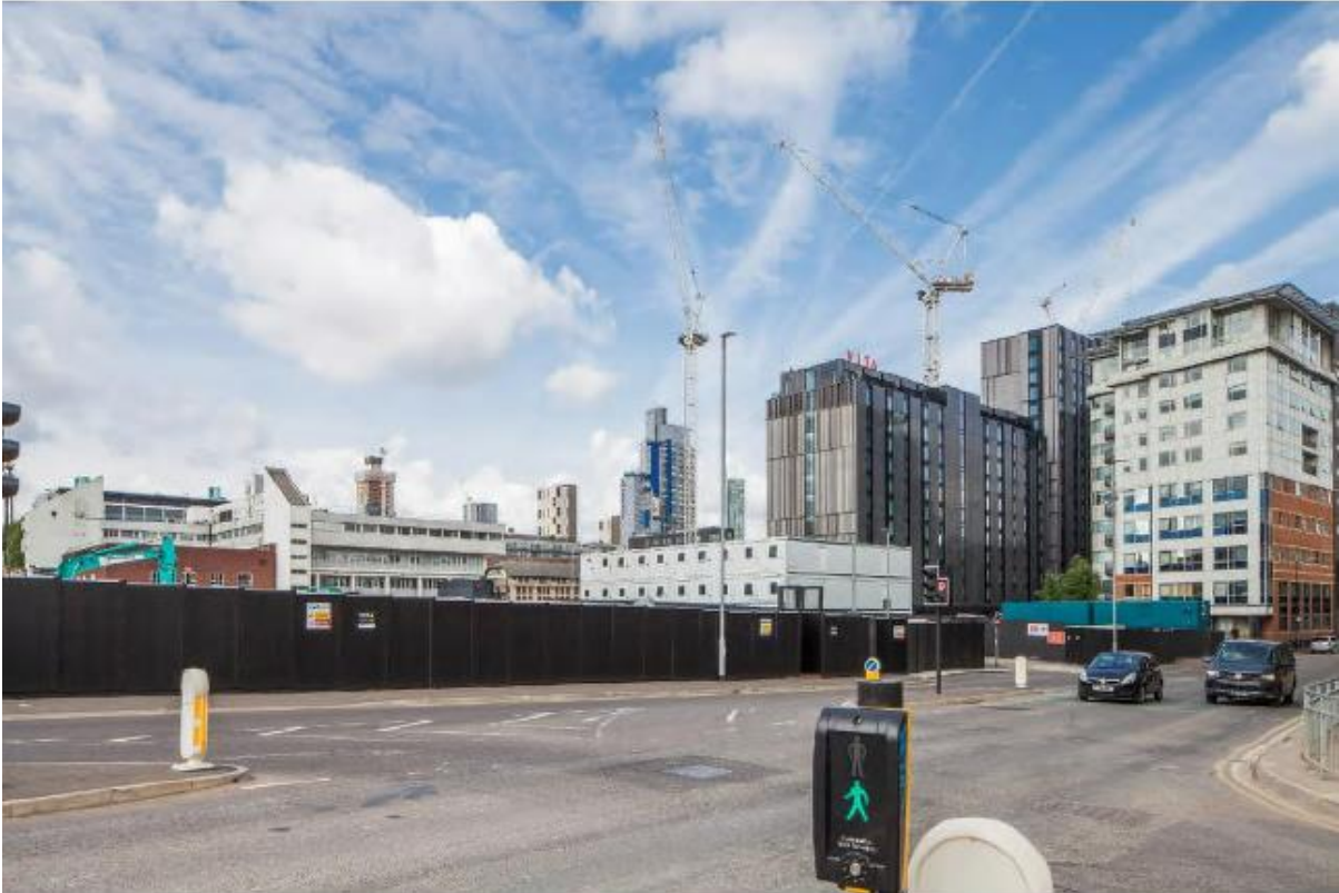
Viewpoint 11 – Brook Street (existing)
